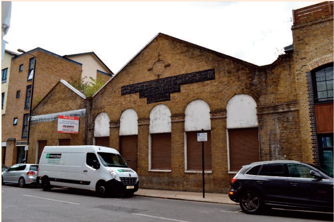
Figure 3: Site A – retained frontage on Wapping High Street
