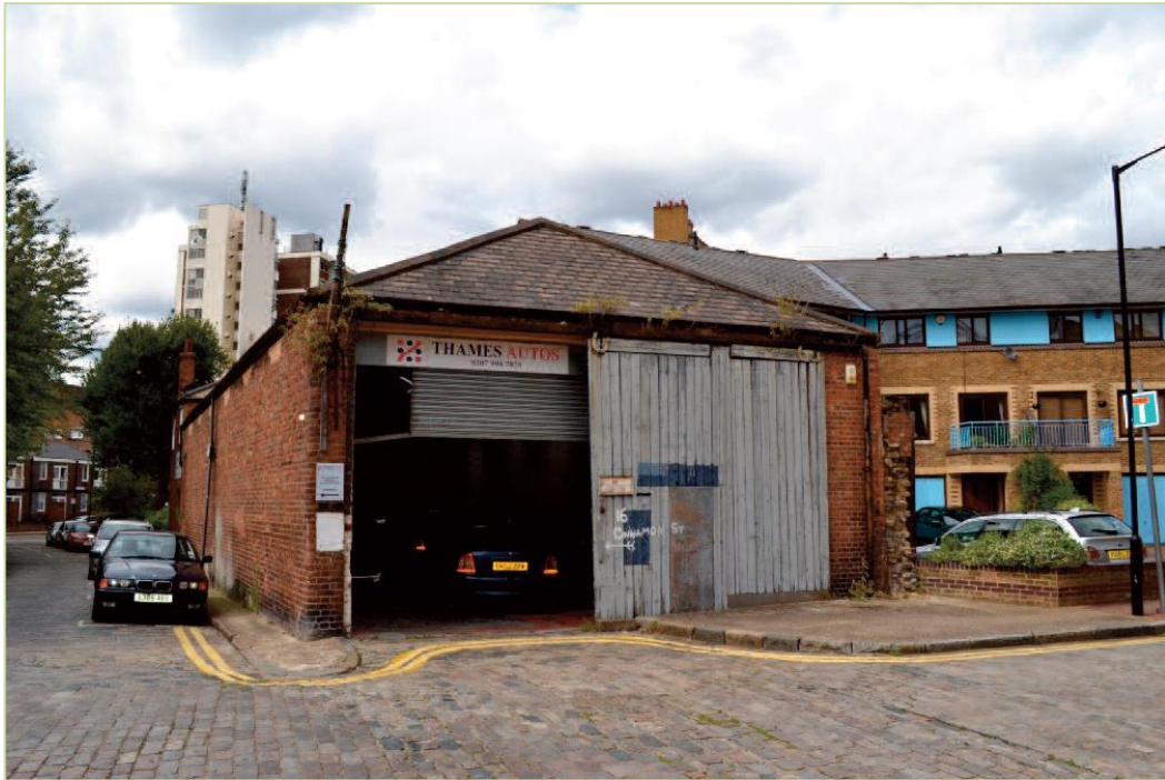
Figure 10: Site C – building used as a garage
